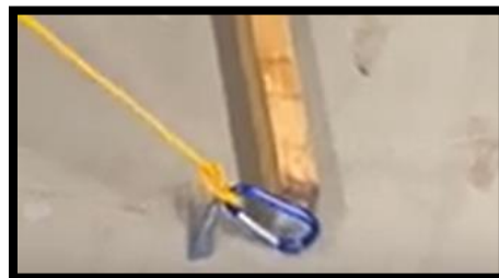
Figure 16 - A Clip Attached to the Rope Connecting to the Hook.
